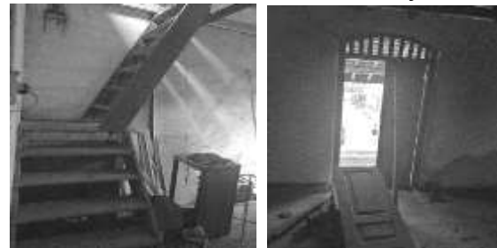
Figure 2: The ladder- like staircase, Source- Author Figure 3: Upper Floor, Source- Author
