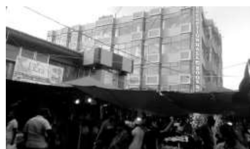
Figure 23- Bazaar Street- Block 2
