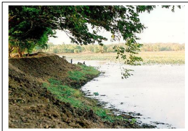
Figure Repaired tank bunds of Ihalakagama wewa Source – K.M.I. Swarnasinghe,2004
